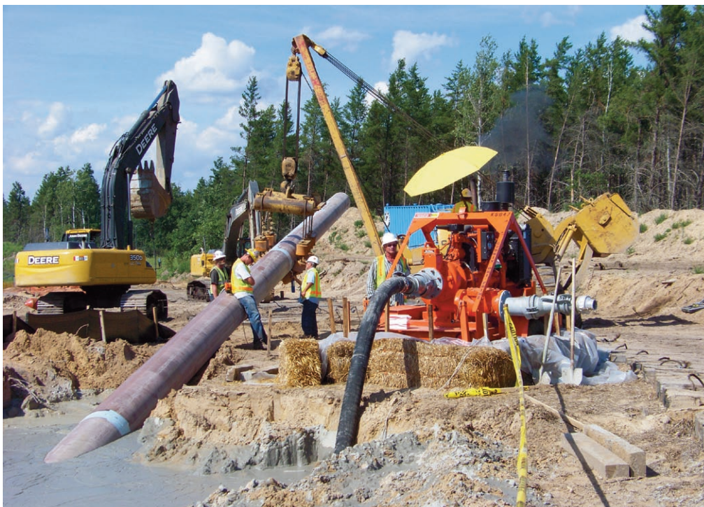
Figure 3. HDD was used to route the pipeline under numerous wetlands.
