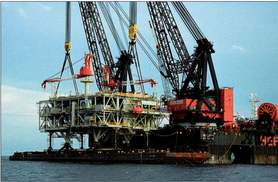
A single-lift deck design saves time and reduces safety exposure.
