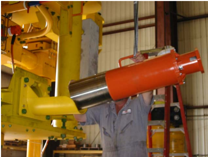
Figure 10: Chemical Metering Valve being Installed
