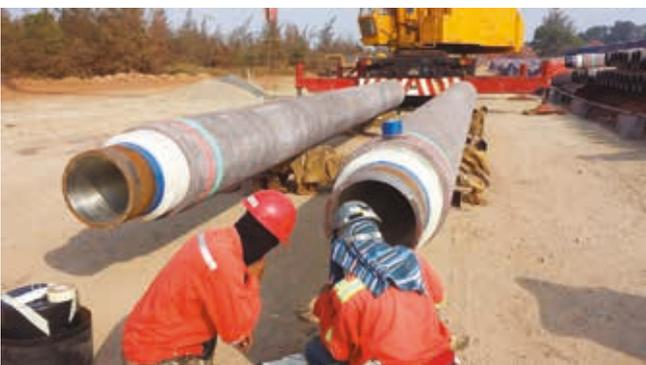
Figure 3. Inspection of concrete and insulation coated CRA clad joints at the coating yard for internal preservation and residual magnetism.
