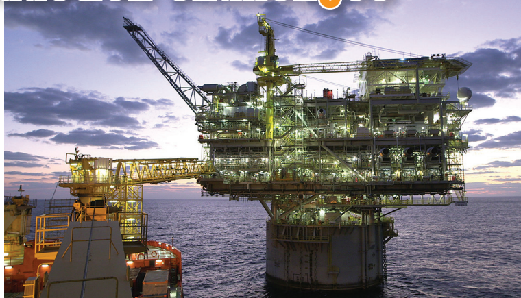
The Anadarko-operated Lucius truss spar, which is operating in approximately 7,100 ft (2,164 m) of water in the Keathley Canyon area in the GoM. (Photo courtesy Anadarko)
